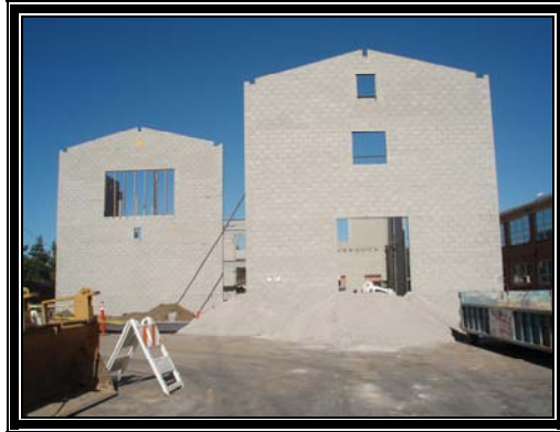
View of the new building from Alonzo Ave.
